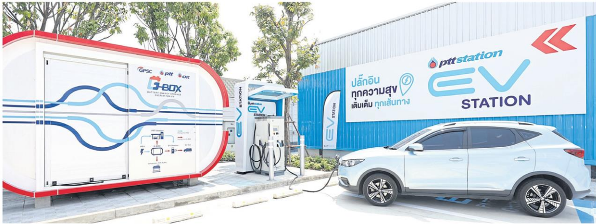
G-Box, an energy storage system that works in tandem with EV charging outlets, was introduced at the PTT station in Bangkok's Nong Khaem district in February this year.
